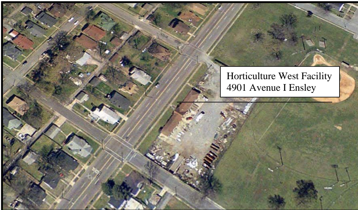
Figure 7-1: Landscaping Chemical Storage Facility
