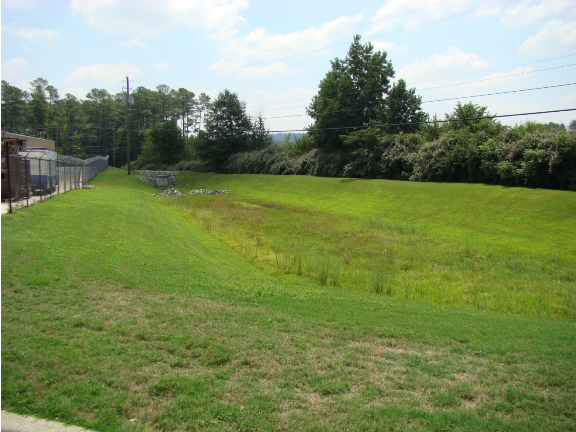
Figure 5-5: Detention Basin in the Oxmoor Industrial Park
